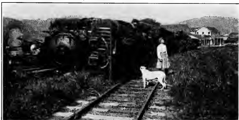
FIG. 293. — Train overturned during the California earthquake of 1906. (Gilbert, U. S. Geol. Survey.)
